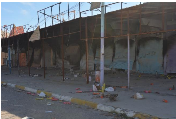
JCC Photo 13: local shops burnt
