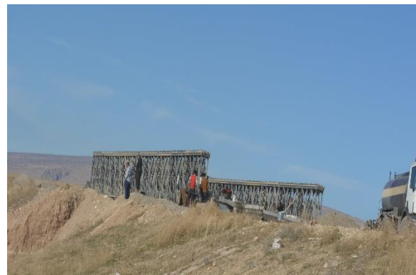
JCC Photo 5: new bridge being constructed on main road
