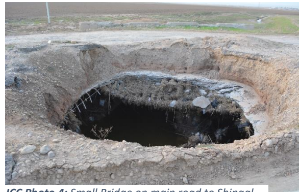
JCC Photo 4: Small Bridge on main road to Shingal
