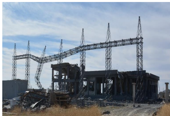
JCC Photo 8: New transformer plant- destroyed
