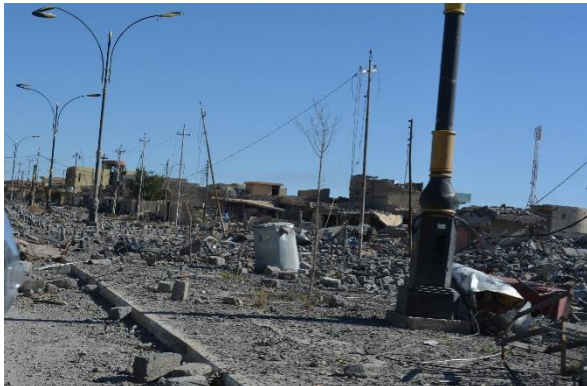
JCC Photo 12: local houses damage
